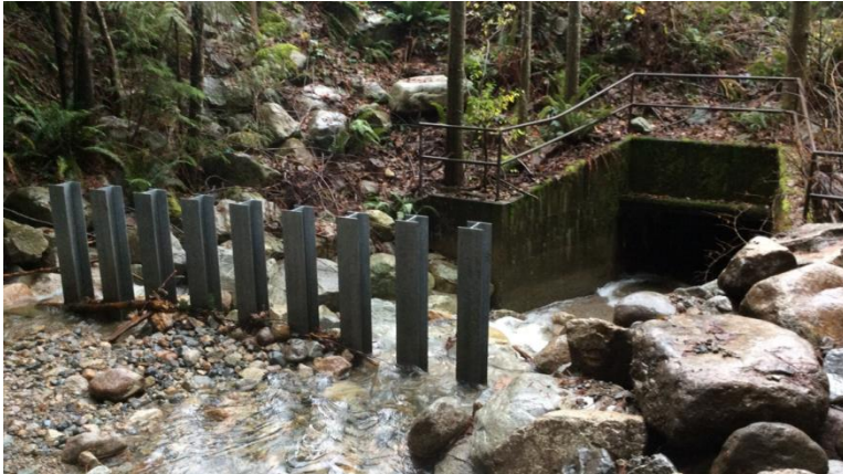
Debris Control Structures
