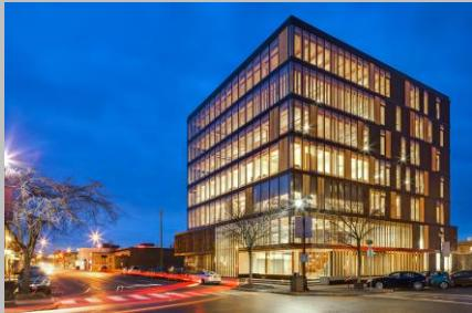
The **Wood Innovation & Design Centre** (WIDC) in Prince George, BC was completed in 2014.<sup>35</sup> The building incorporates a structural system that includes a variety of solid engineered wood products including CLT, glu-lam and LVL.
