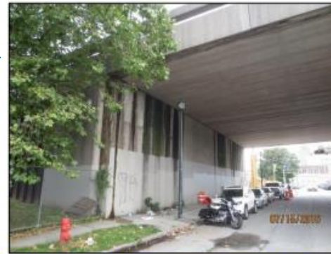
West abutment with stains from water leaks.
