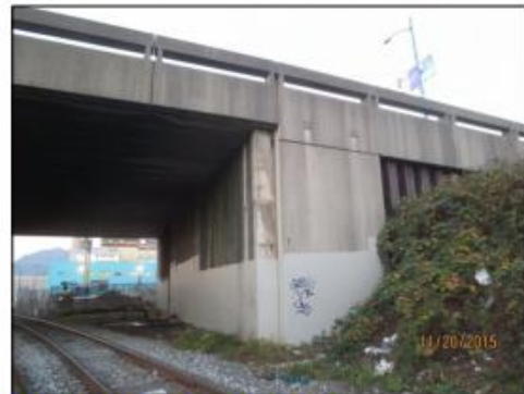
South corner of east abutment.
