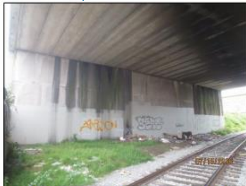
East abutment with stains from water leaks.
