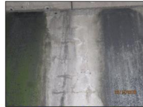
Existing vertical cracks in west abut concrete.
