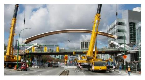
Kingsway Bridge, Burnaby, BC. Spanning 145 feet across a major arterial roadway, Kingsway Pedestrian Bridge's one-of-a-kind construction consists of a timber-steel arch with the post-tensioned segmental precast concrete walkway acting as tension tie. Source: Fast+ Epp
